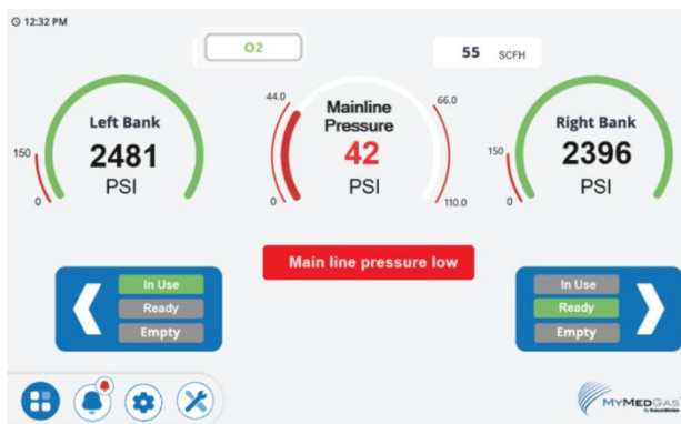
Figure 23 - Low Line Pressure Fault.
