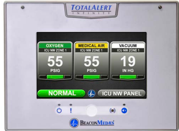
Figure 59: Area Alarm User Interface
